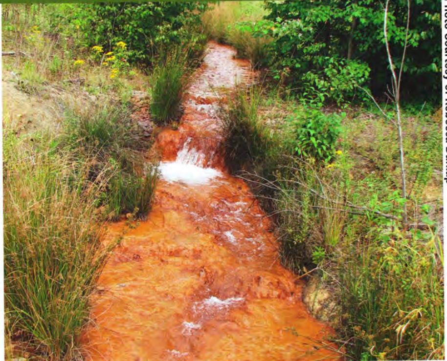
SULFUR CREEK White Oak deep mine discharge near Madera, PA
