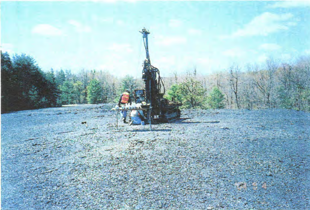
Figure A-43. Coal Refuse Bank RB-1 with Auger Drilling Equipment.
