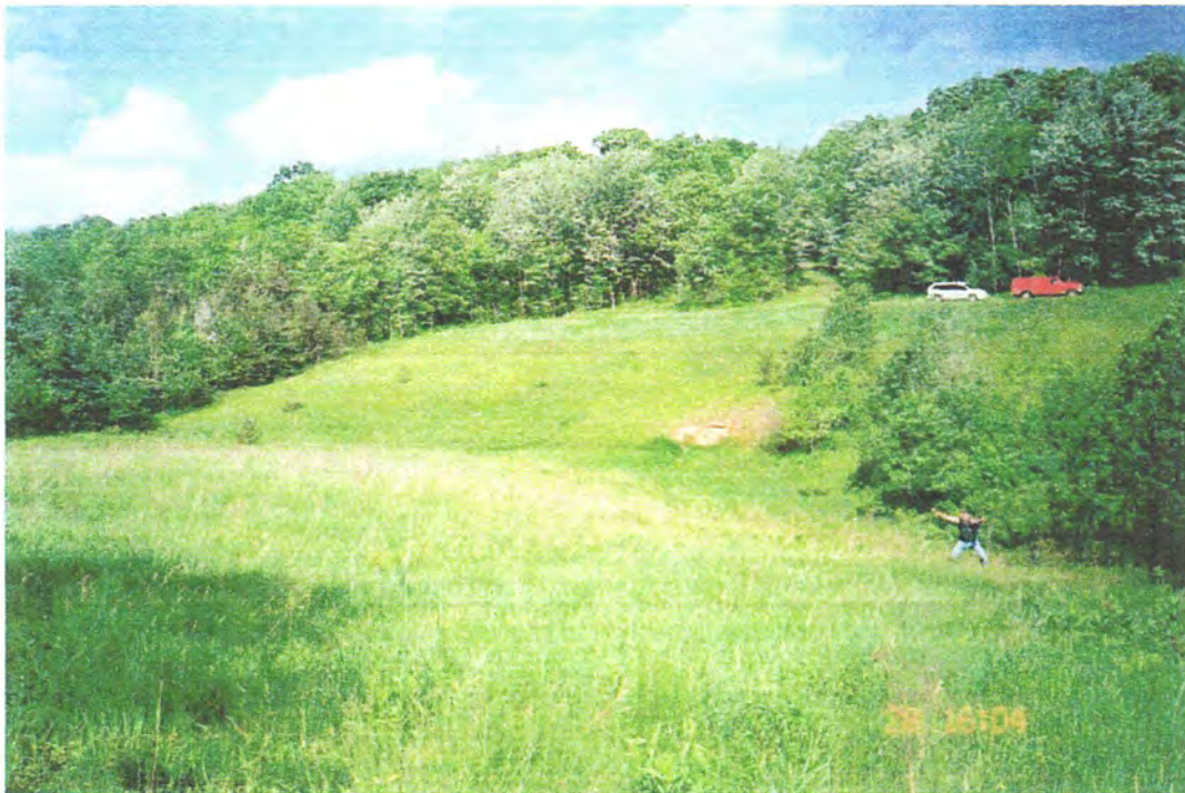
Figure A-37. Reclaimed Brookville Mine Area SM-12A with Collapsed Deep Mine Entries.
