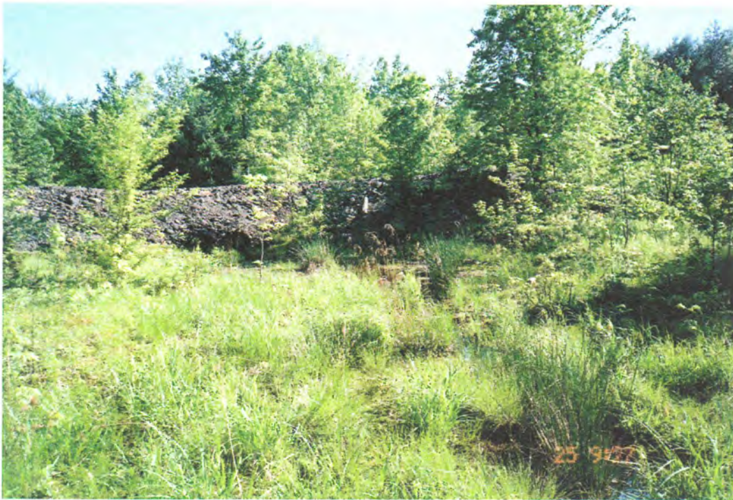
Figure A-47. Coal Refuse Bank RB-2 from the Contrary Run Valley.
