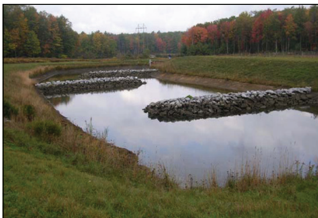
Pine Glen East passive treatment system in the Boake Run watershed.
