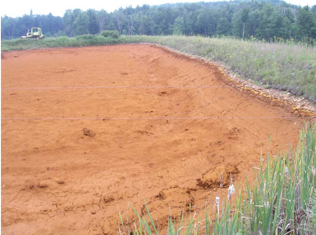
Figure 2. Iron accumulation on bottom of VFP1 after draining for rebuilding. But the pond was flowing through this without overflow.
