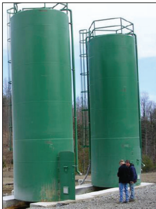
Lime dosers in the Dents Run watershed.
